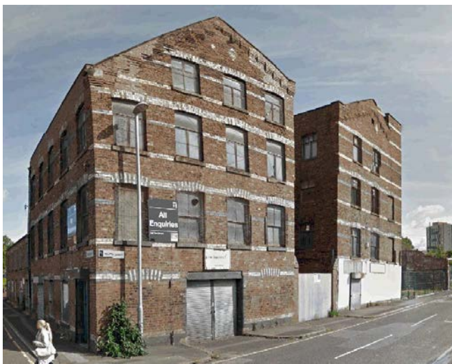
The building on the left (107 George Leigh St to be retained) All other buildings proposed to be demolished
